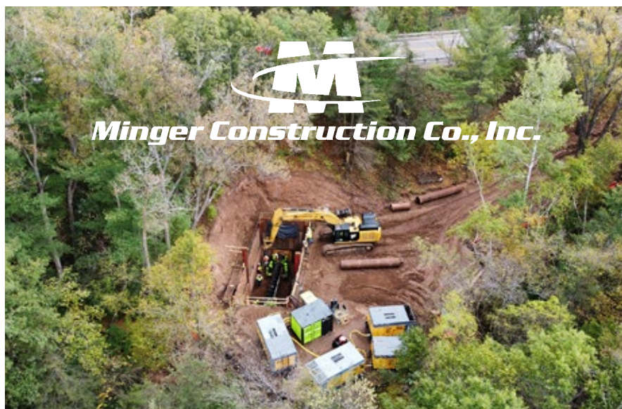
AFTER: A pile of cuttings generated during installation by the horizontal down-hole hammer boring process
