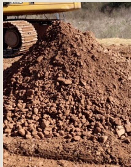
AFTER: A pile of cuttings generated during installation by the horizontal down-hole hammer boring process
