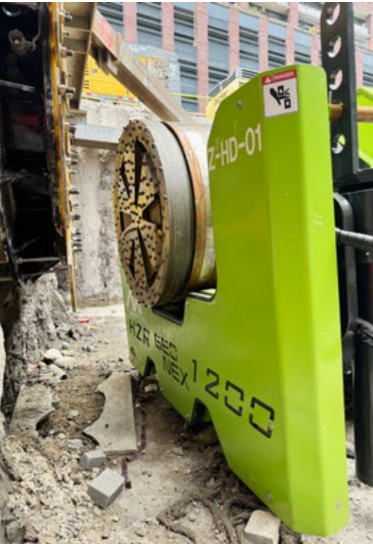
The face of the boring system used to pulverize the rock
