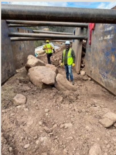
BEFORE: A worker stands next to boulders retrieved during excavation of the launch pit
