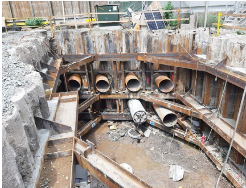
Receiving pit – showing 6 of the 8 completed installations using the DTH method
