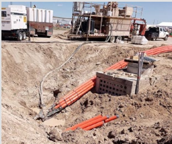
Very busy summer installing multiple bundles of 4-inch conduits
