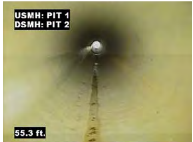
Left photo shows 12-inch CML-lined cast iron pipe post-cleaning, preparation and pipe drying with airborne stone. Right photo shows the pipe (at the same location) after CIPP lining.
