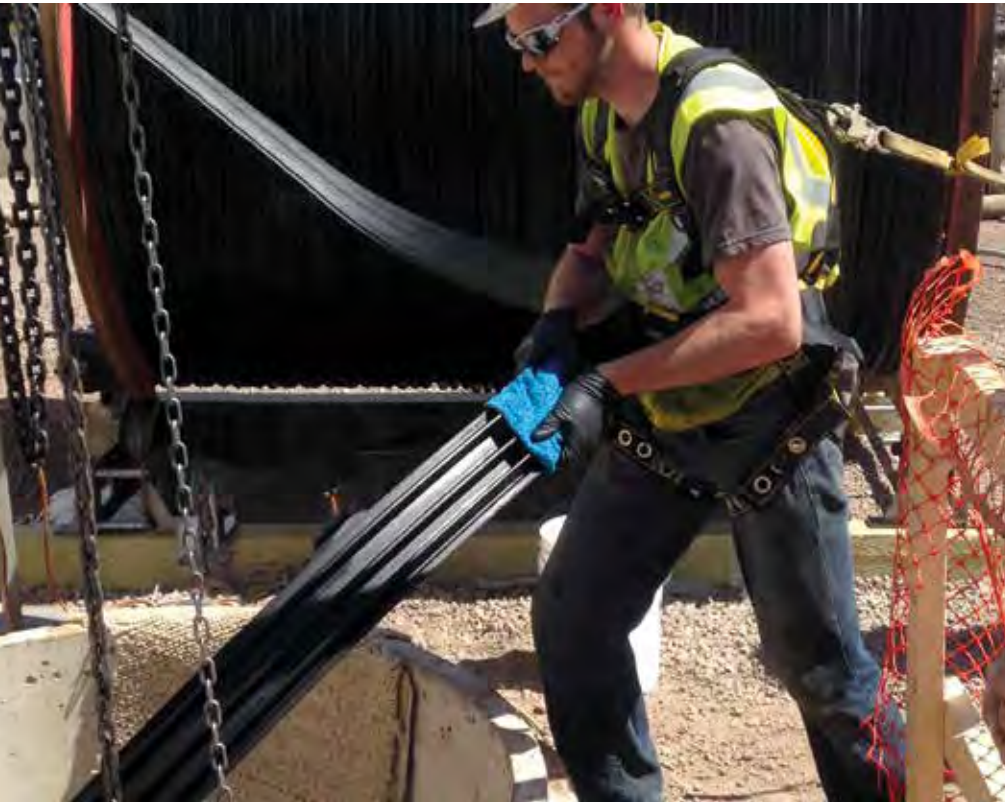
A single strip of steel reinforced HDPE profile was progressively fed into the winding equipment inside the existing pipe
