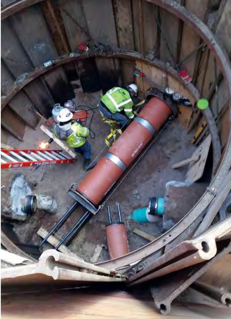
Minger Construction used a variety of shafts at depths of up to 20 feet
