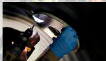
Anchor installation onto the brim through the steel ring
