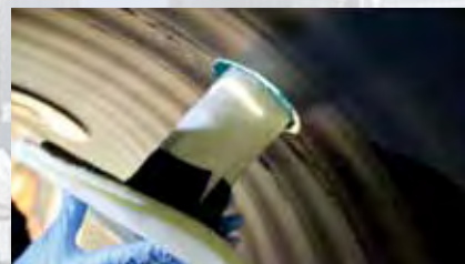
Lapel Liner inserted into service line
