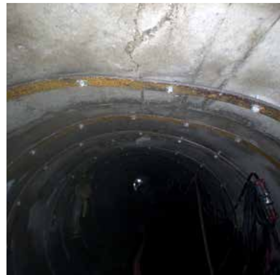
Structural steel banding was placed in the crown of the RCP in order to allow for safe work activity inside. The crown and invert had cracked due to excessive loads.
