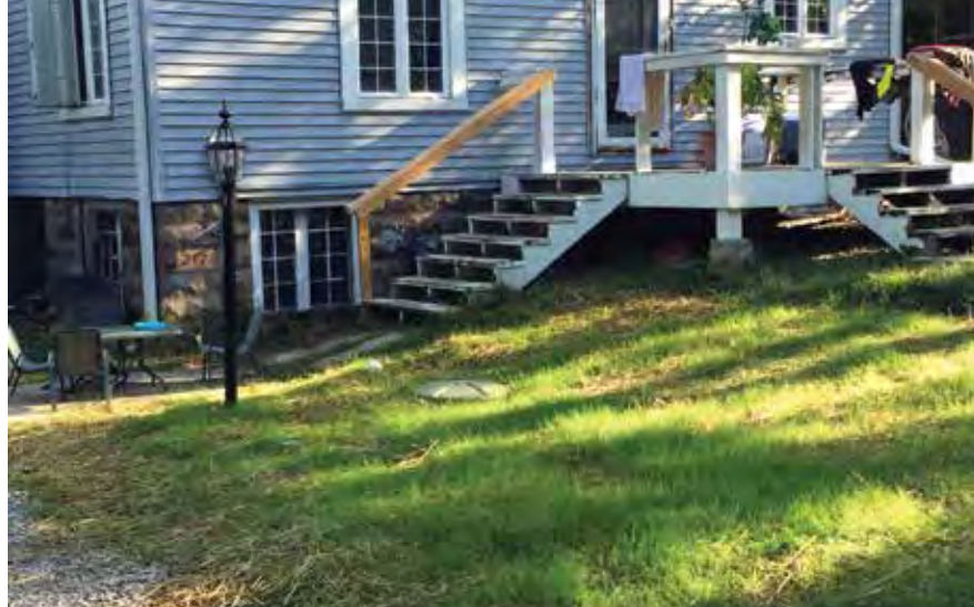
Post installation. Grinder pump lid is low profile, approx. 2 inches above ground
