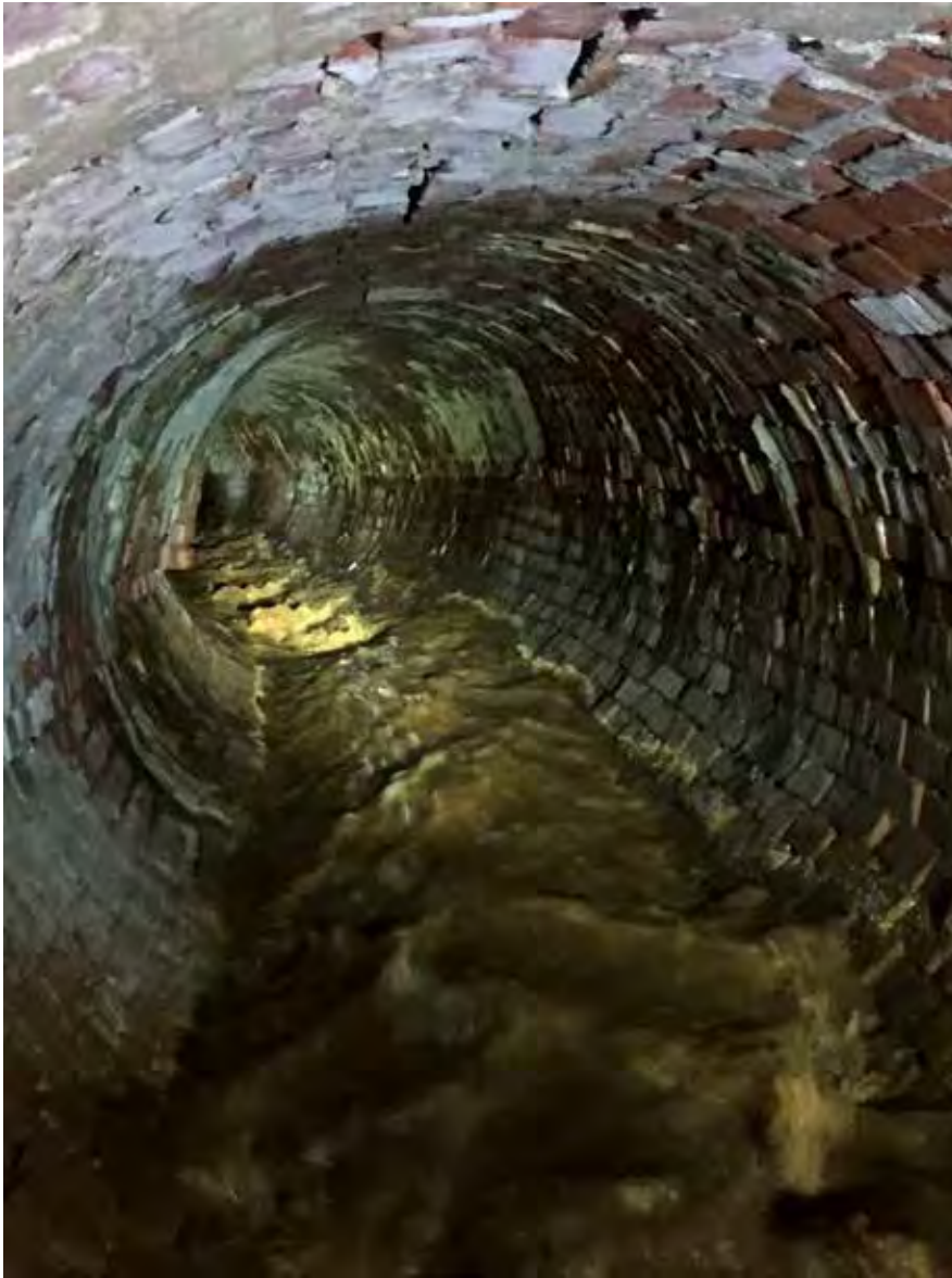
Original brick sewer showing curved section
