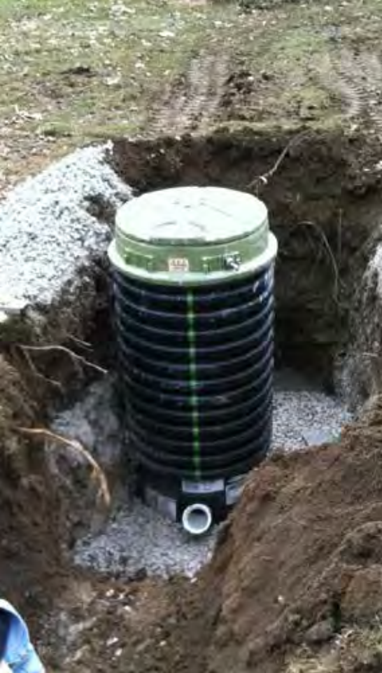
New grinder pump in place
