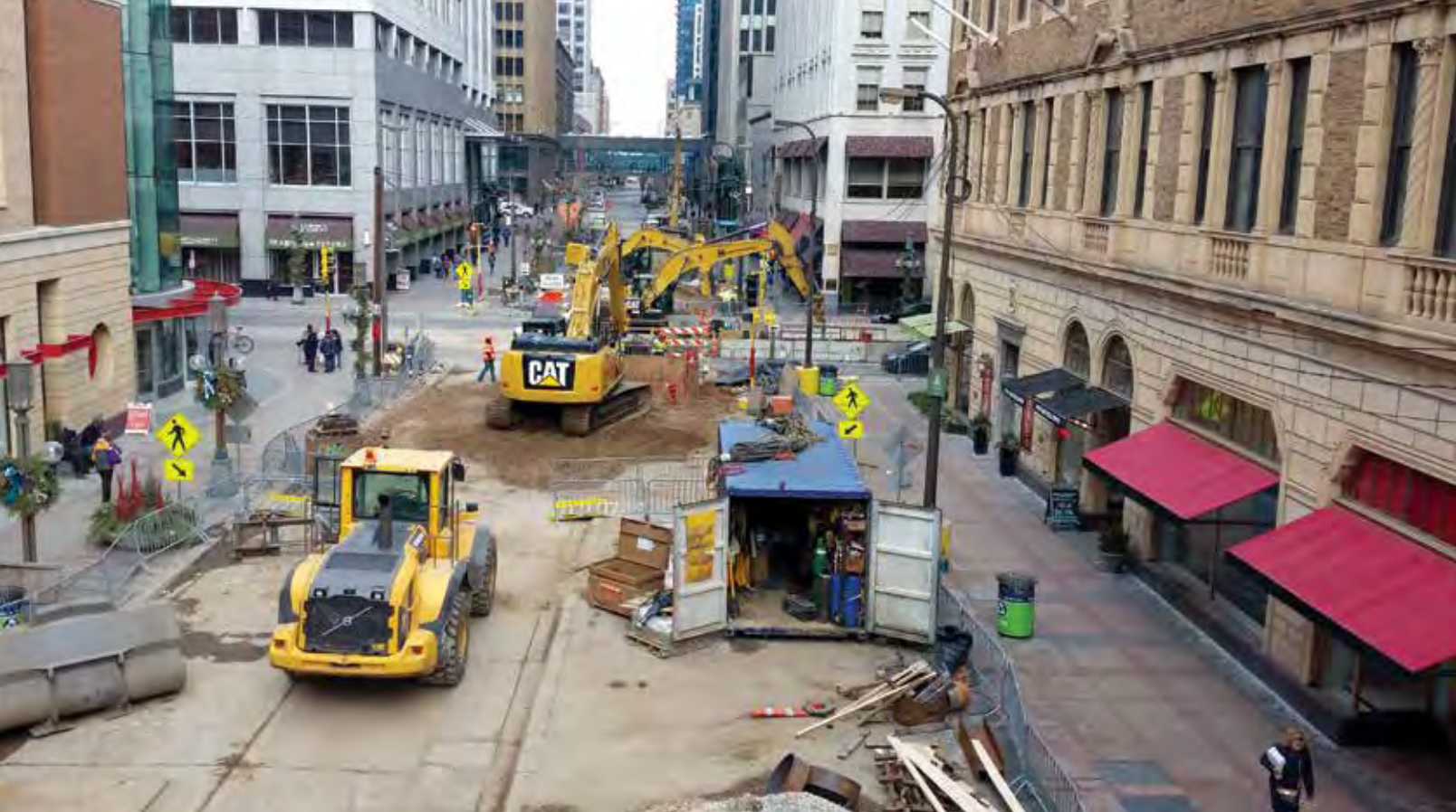
Tight working conditions in active urban areas make trenchless installation using the Pilot Tube Method the best option.
