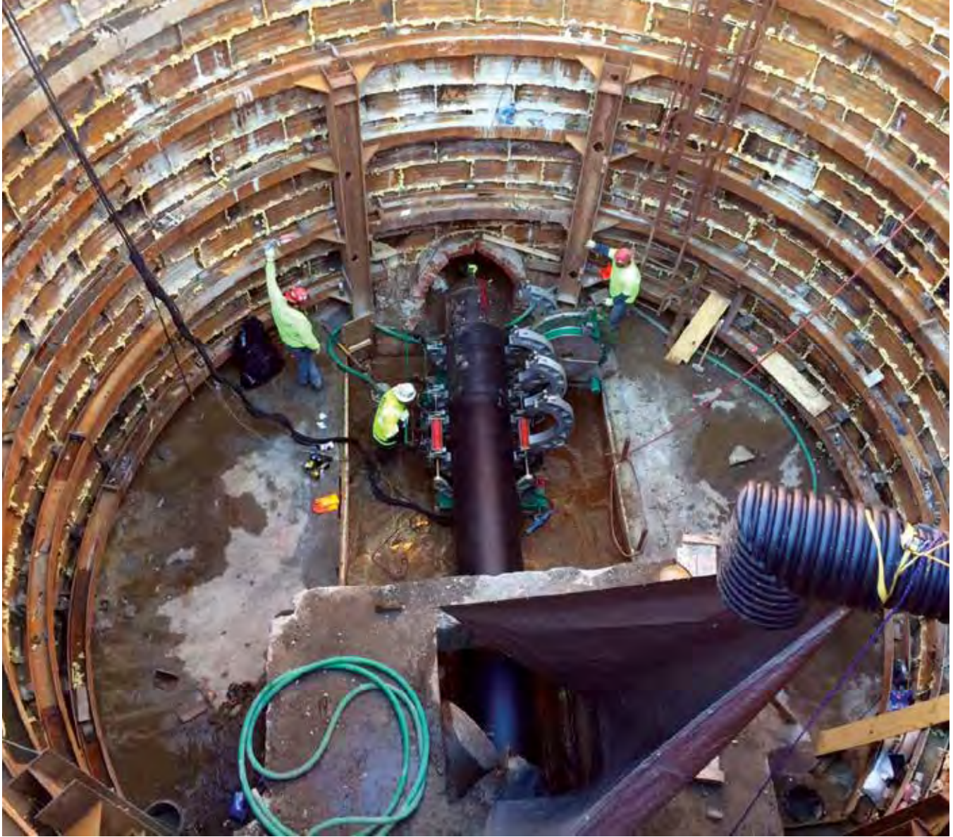
Installing HDPE pipe proved to be a well thought out and wise solution
