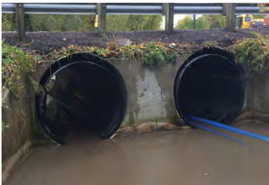
Helically wound Smooth Cor™ is sliplined into the existing host pipe
