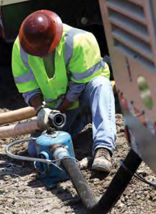
The ramming tool is lubricated during operations, inline, with a specially formulated lubricant designed for pneumatic tools that does not deteriorate air hoses or plastic pipe
