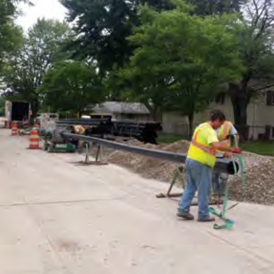
Pipe Welding Set Up, Bloomfield Orchards, MI
