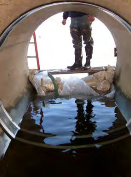
Installation of the HydraTite® Internal Joint Seal was accomplished in less than an hour by two technicians
