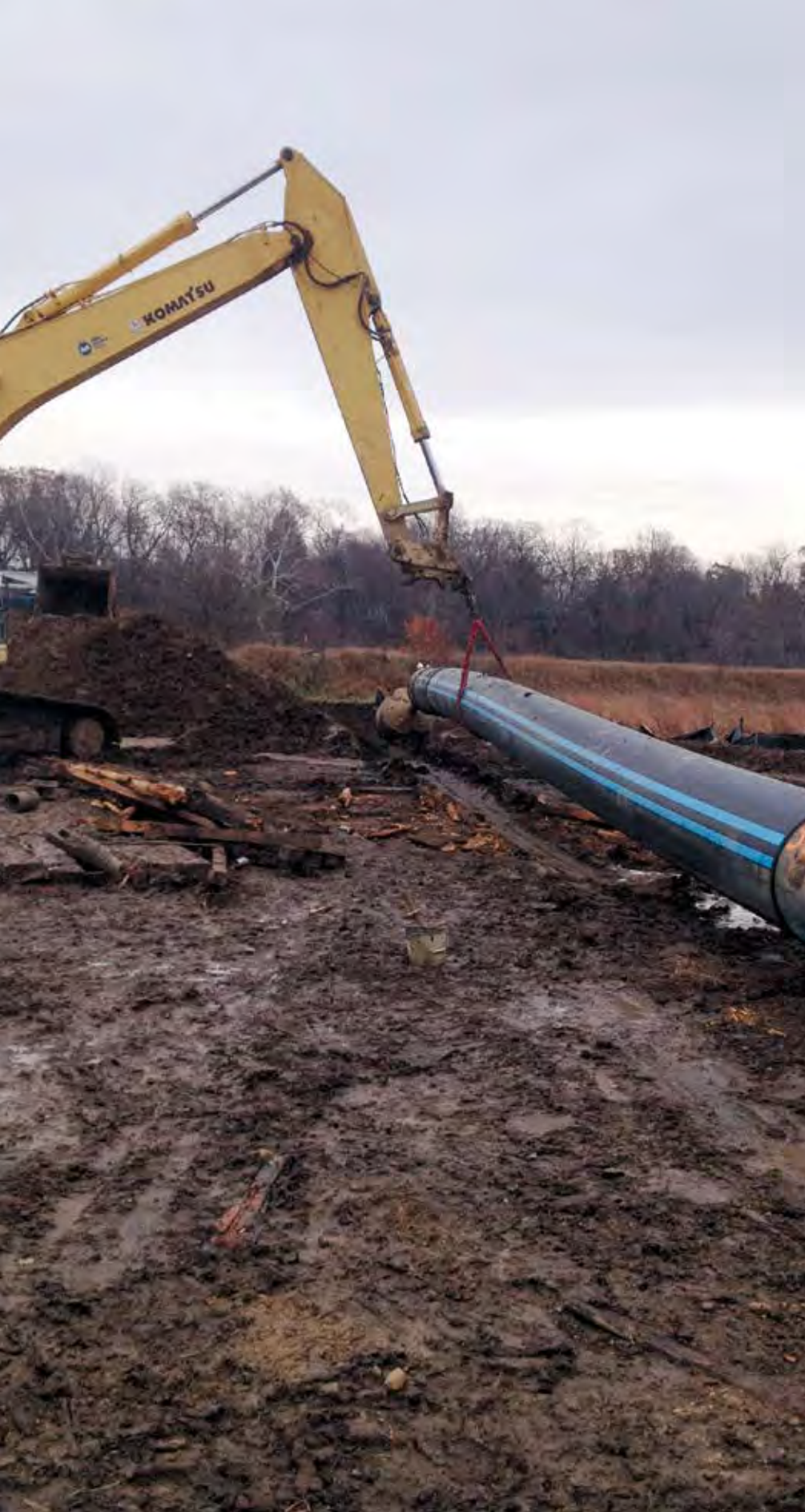
1,100 feet of 30-inch diameter solid wall HDPE was used
