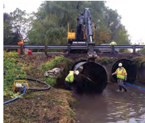
The longer lay lengths made it easy to insert the Smooth Cor™ pipe using a smaller equipment
