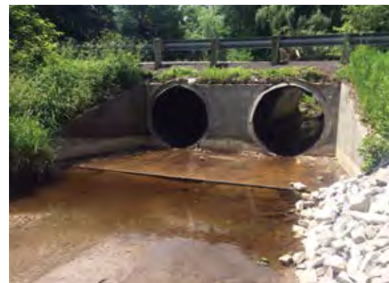
Completed Smooth Cor™ reline project extended the service life of the original culverts
