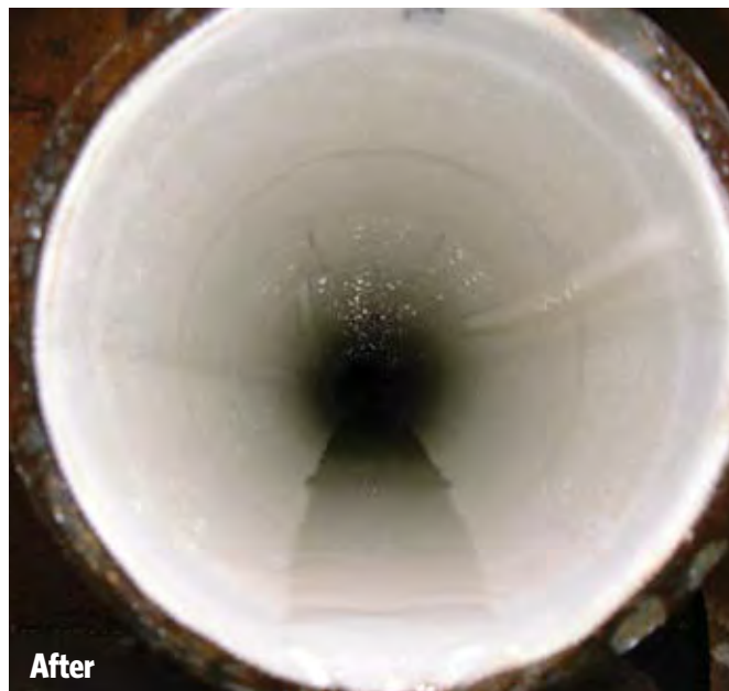
Epoxy migrates through the outer jacket of the liner to fill all voids around the services and any existing spaces within the host pipe, creating a full bond to the interior of the old water main
