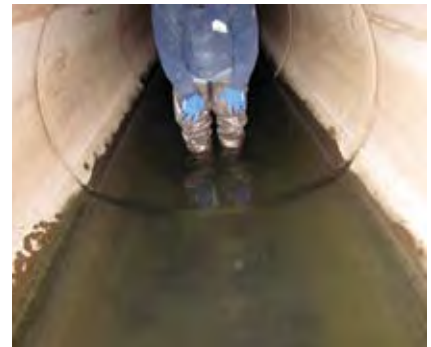
There was approximately 18" to 24" of standing water in the pipe
