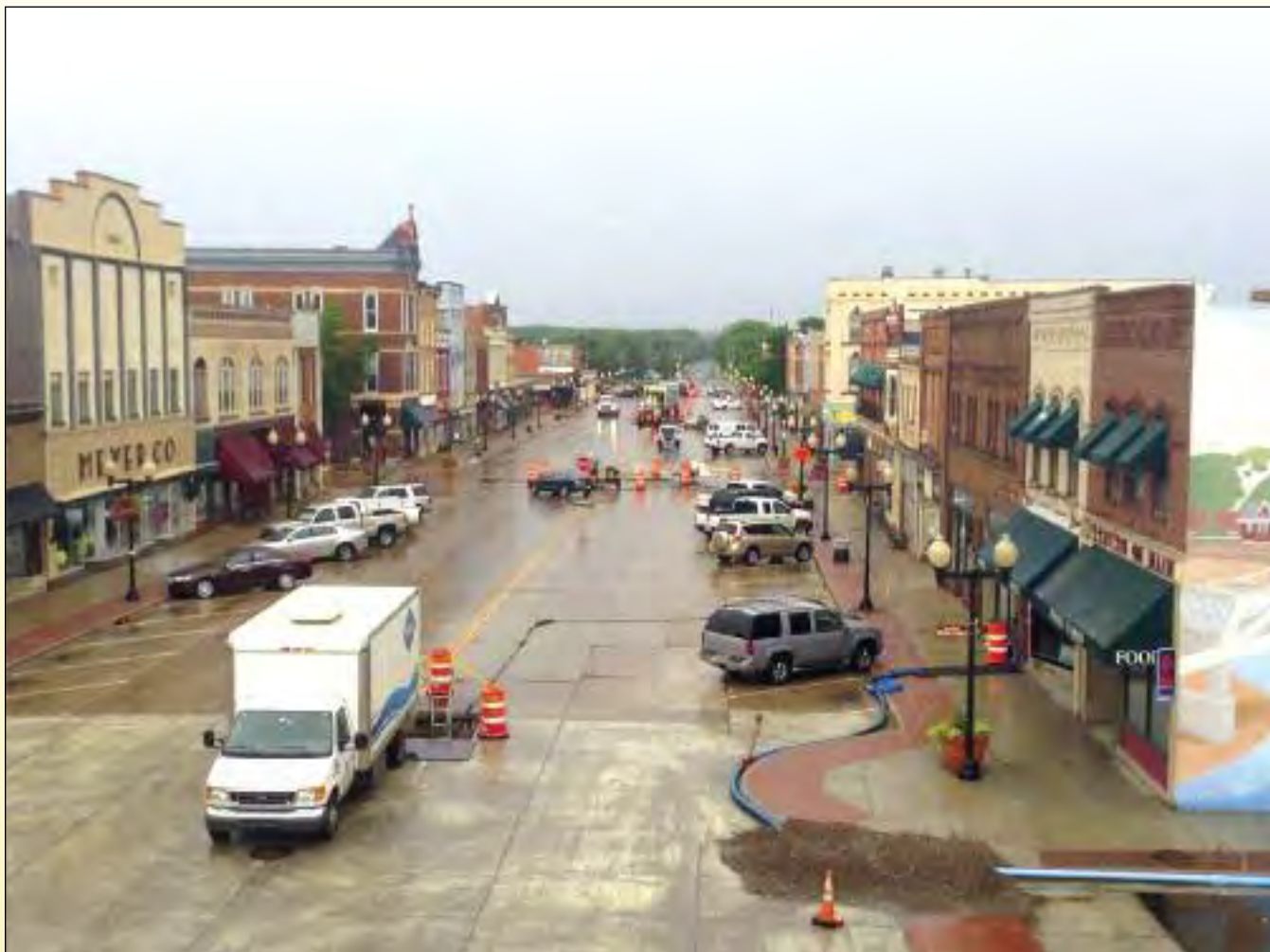
Lining was installed via 12 small pits located in the middle of the street.
