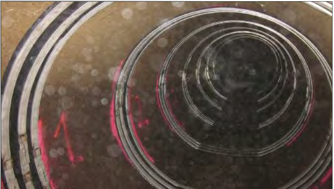
The first three bands were assembled at the pipe joint and then placed into the seal after it was opened and positioned. The other four seals were installed after the bands were assembled in the manhole and then moved into their proper location at each joint.
