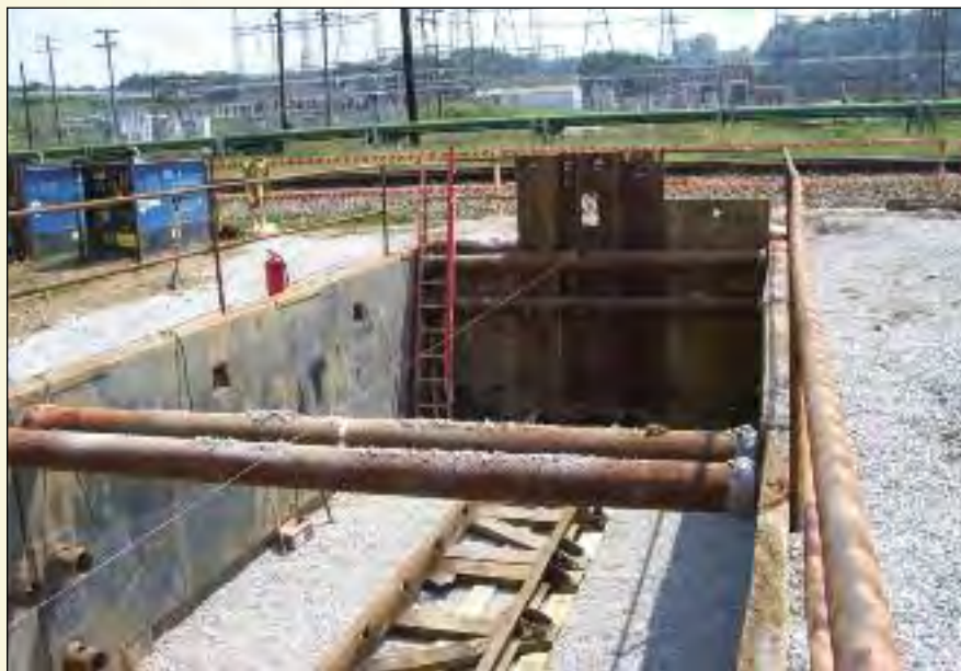
Figure 2. Trenchless Launching Pit Installation for Crossing Railroad
