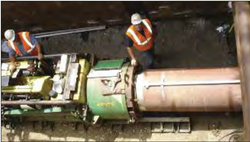
Jacking the 30-inch VCP in the final step was the smoothest part of the installation.
