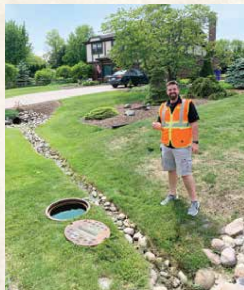
The first T-Liner revisited 23 years later by Robinson Engineering, Ltd. & Performance Pipelining, Inc.
