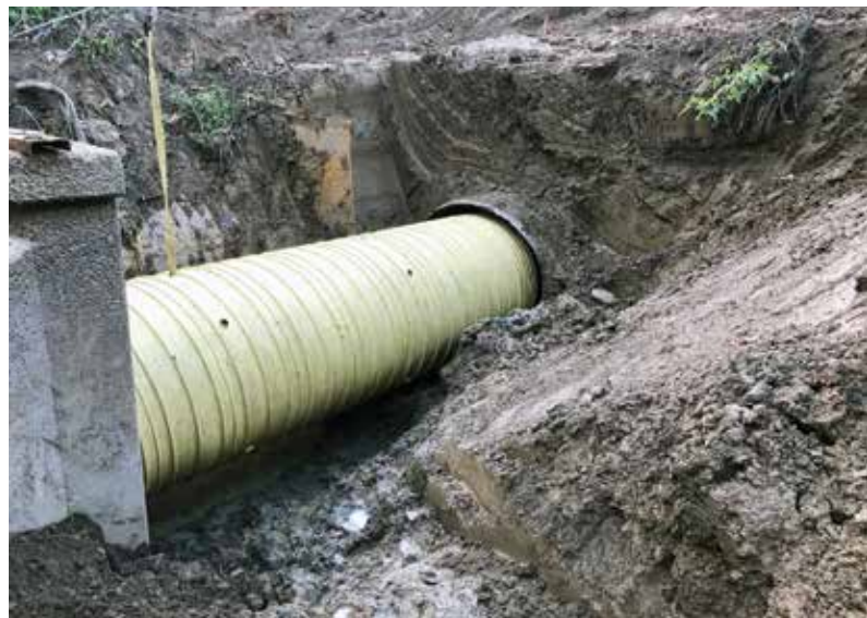
The liner pipe is inserted into the host pipe utilizing a push/pull method
