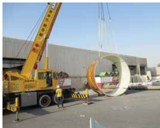
Proprietary system offered a way to break the geometrically complex pipe liners down into multiple component segments to dramatically reduce shipping costs, while still maintaining structural integrity and load capacity
