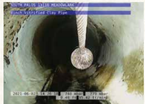
The first T-liner, mainline piece only slightly visible under a subsequent mainline CIPP installation
