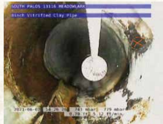
A golf ball sized hole in the first T-liner where a mainline lining company gouged too deep during service lateral reinstatement
