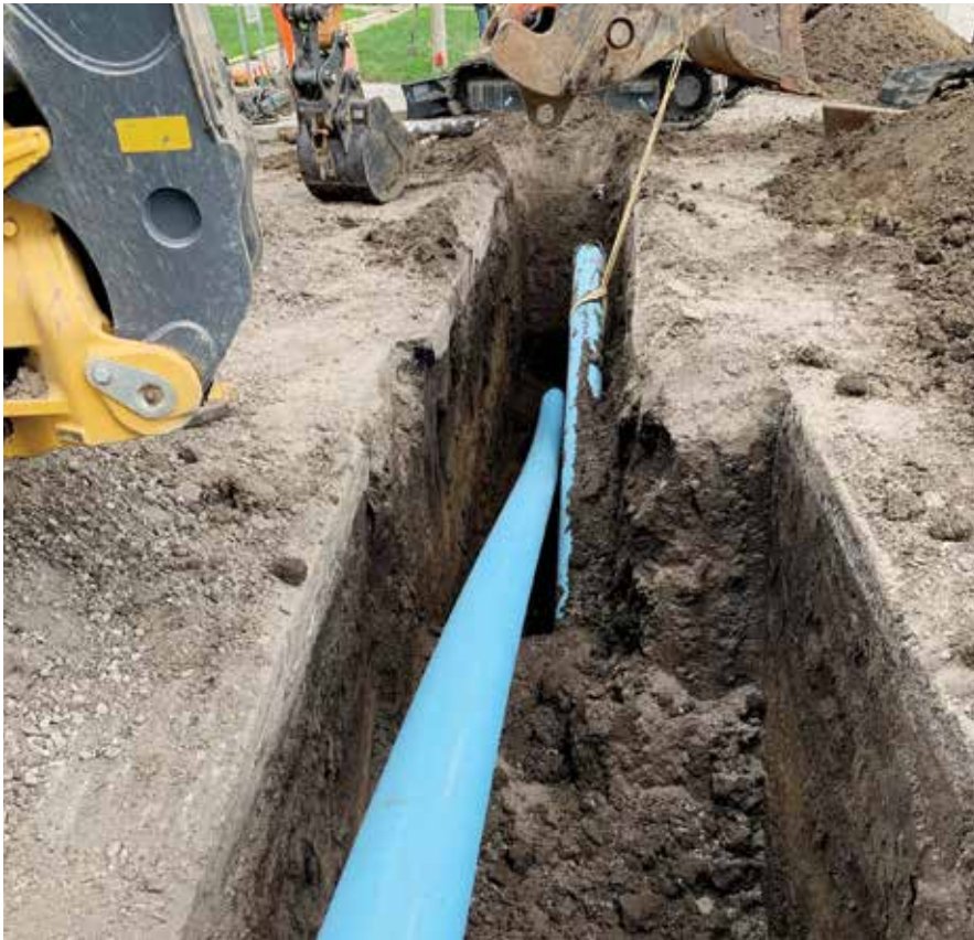
Over several pipe bursting projects, Basaraba has used restrained joint PVC, fusible PVC and poly. One the benefits of static pipe bursting is the method's ability to use a variety of product pipes
