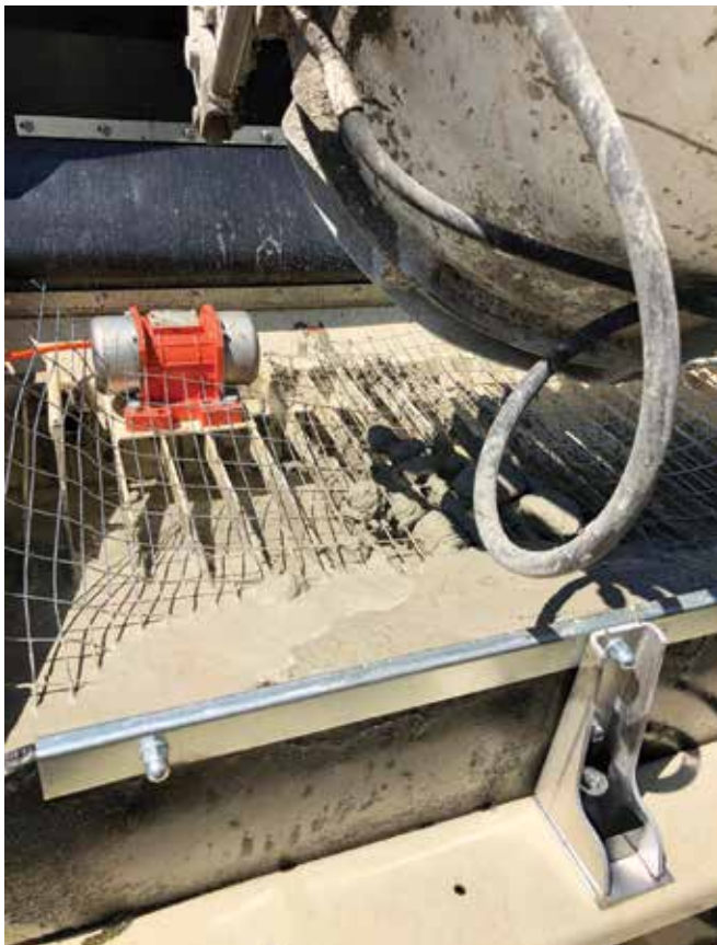
A screen on the pump hopper should always be used to sift out any large aggregate that can clog the grout line and potentially damage the structure
