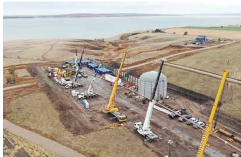
On October 23, 2021, the HDD and pipeline crews successfully worked together to pull the 24-inch welded steel pipe through the reamed hole, completing the crossing
