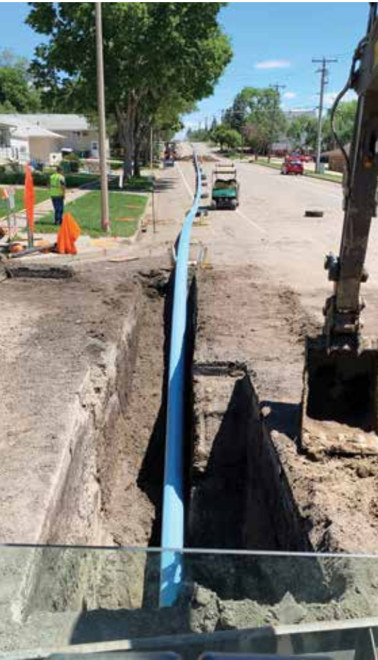
Basaraba crews try to complete 800 feet of bursting per week, start to finish. Since starting pipe bursting work, Basaraba's Excavating and Dirt Works now focuses almost exclusively on trenchless
