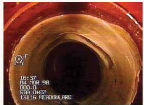
The first T-liner, mainline piece at time of original installation
