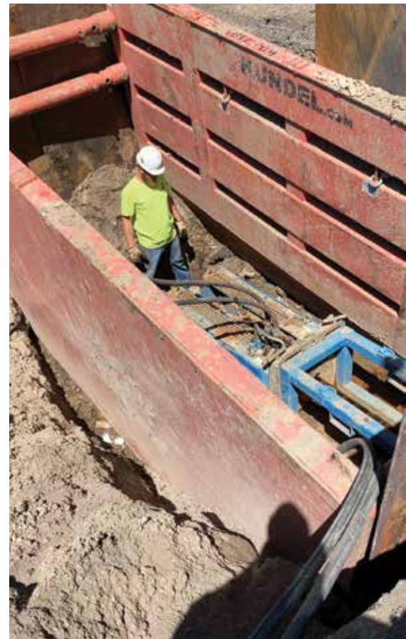
Basaraba's first bursting project for the City of Bismarck, ND included replacing 8,000 feet of 8-inch cast iron water main to 10-inch Certa-Lok® restrained joint PVC using a Grundoburst 800G static pipe bursting system
