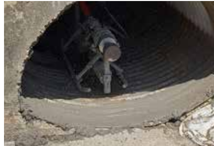
Cement Pipe Rehab
