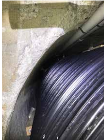
Each piece was moved and blocked along the required 1000-foot length
