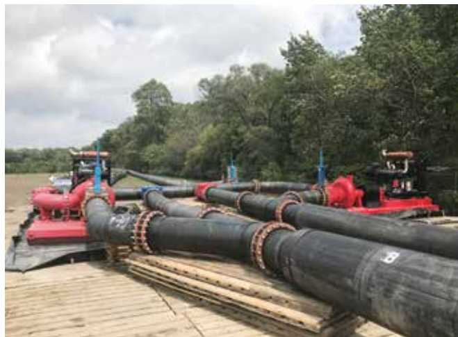
Figure 3. Booster Station
