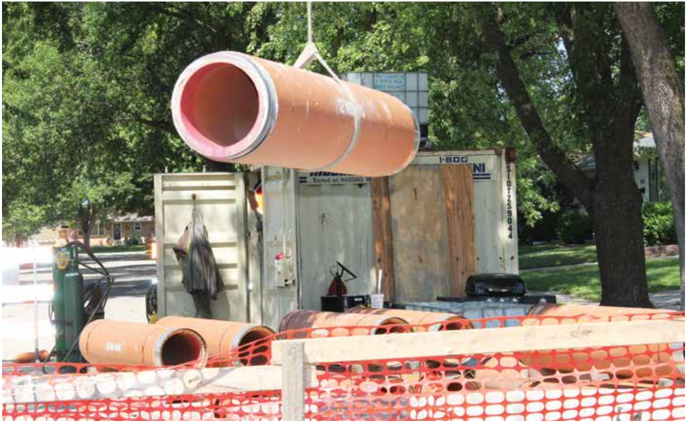
Owner selected pilot tube method to minimize construction impacts for residents. Method also presented project savings because of deep installation of the new sanitary sewer
