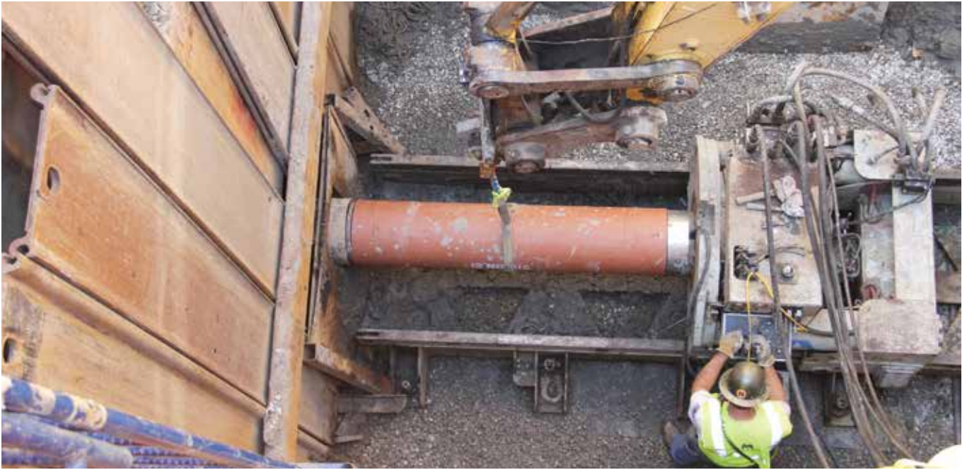
Minger Construction, Inc. installed a new gravity relief trunk sewer at up to 30-foot depths to alleviate capacity during peak wastewater events
