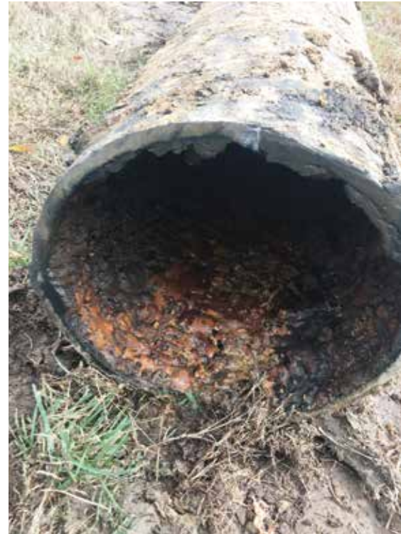
Midwest Mole replaced piping that was 95- to 100-years-old with HDPE. Pipes ranged from 2- to 12-inch diameter
