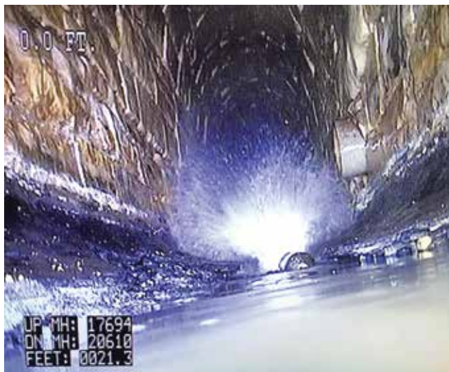
Figure 6. Invert damage caused during cleaning operations had to be repaired with bricks and flowable fill
