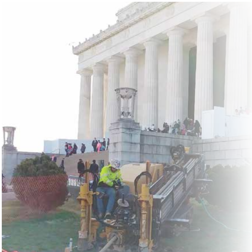
It's not every day an HDD operator can say they worked in front of the Lincoln Memorial
