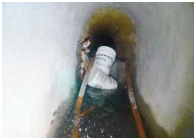
Figure 4. A dam was constructed and used to control flow during bypass pumping operations within the arch sewer
