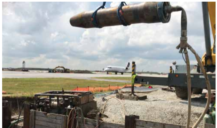
Extensive shoring was required
