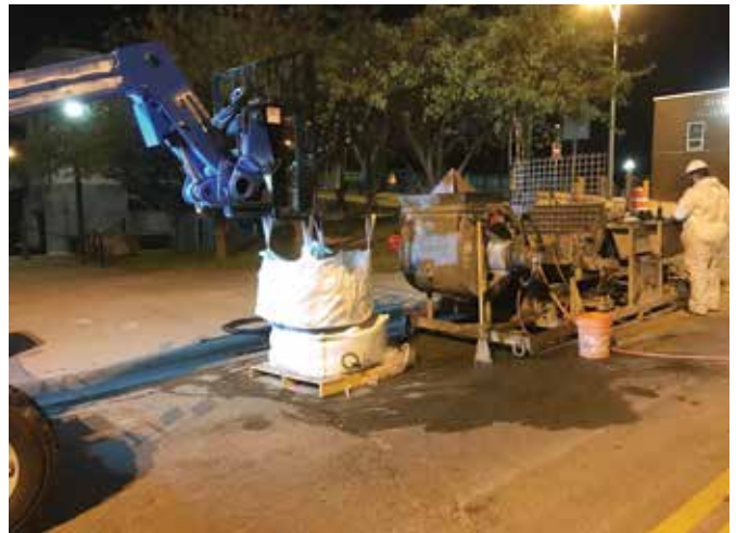
Figure 3. The small footprint of the geopolymer lining operation in a tight downtown business district
