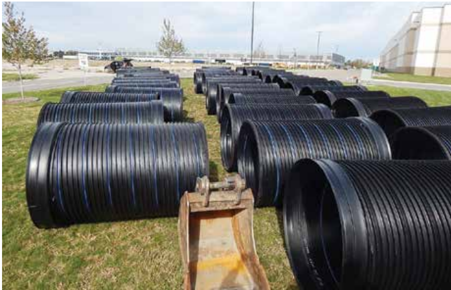
Using shorter pipe lengths eliminated the need for any access pits within the existing storm sewer line
