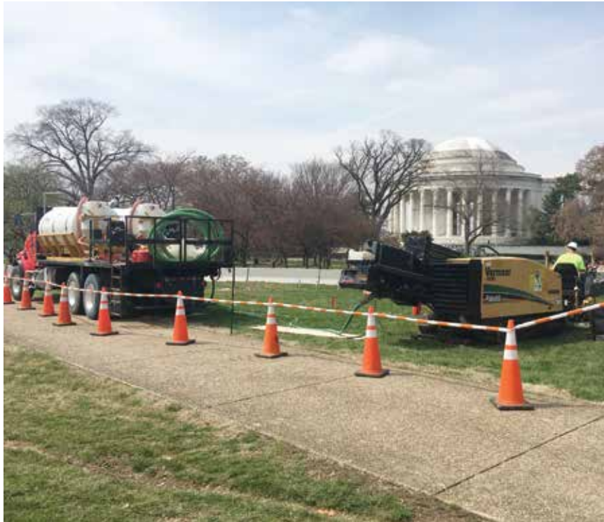
Impressive project was a testament to the less invasive nature of trenchless technologies
