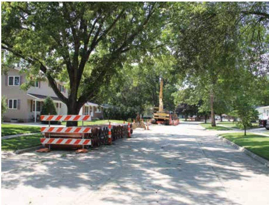
Project location in a residential area, City of Fort Dodge, IA. To maintain accessibility, construction material and equipment had to be staged strategically so that it did not block driveways
