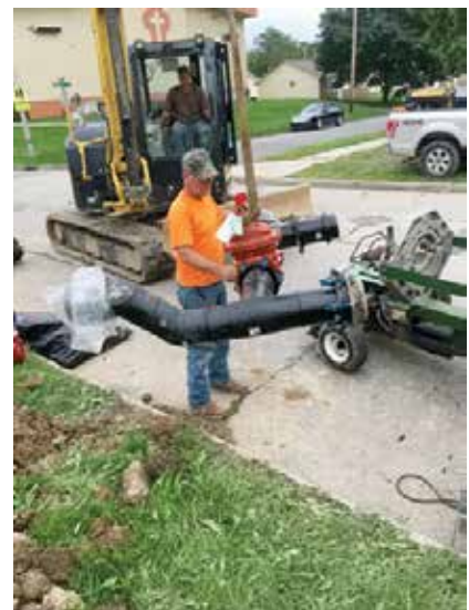
HDD used to install six-inch diameter water main from 500 foot reels. City crews have become skilled with electrofusion
