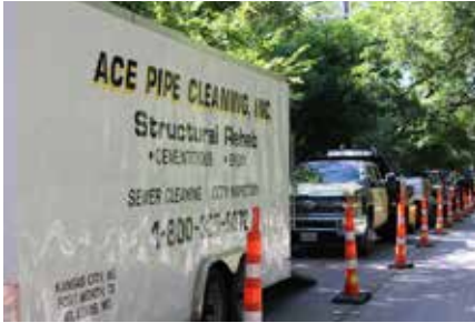
Sewer Cleaning & CCTV Inspection
