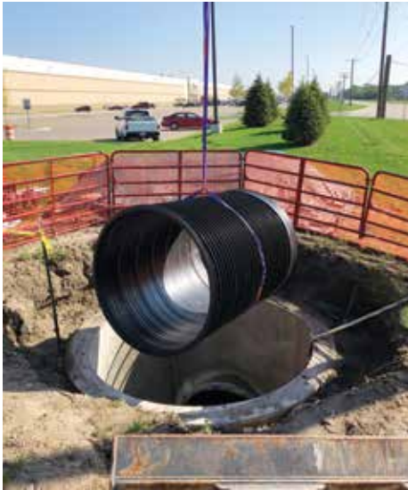
Seven foot lengths of DuroMaxx SRPE liner pipe were lowered into the existing storm system
