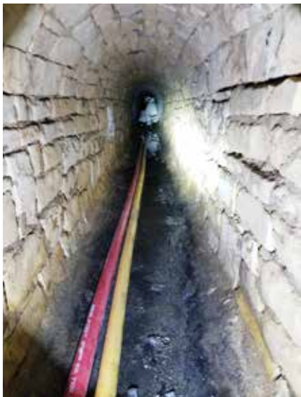
Figure 1. The limestone archway sewer before rehabilitation in the City of Joliet; constructed in the 1860s
