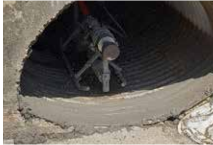
Cement Pipe Rehab
