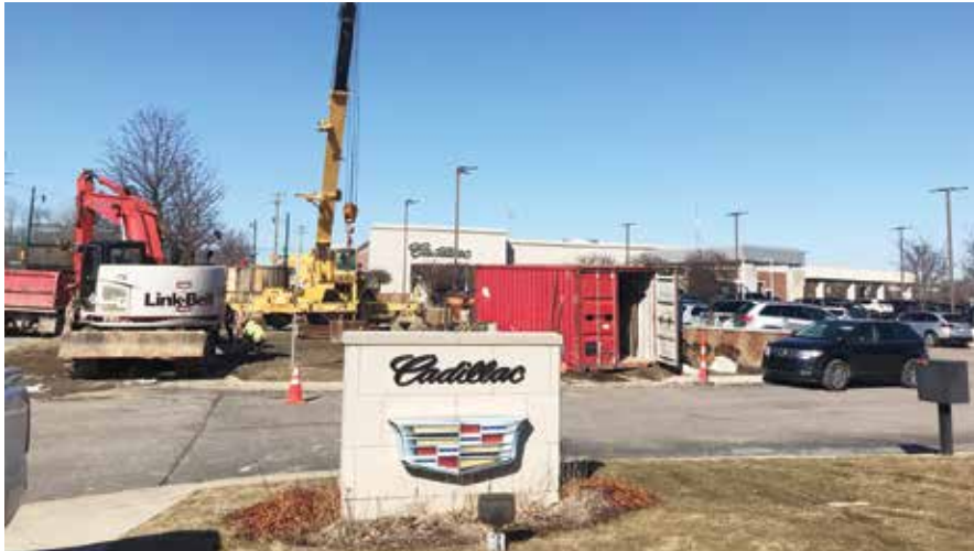
Minimal footprint of PTM construction at the east end of the project minimized disruption to the Cadillac dealership
