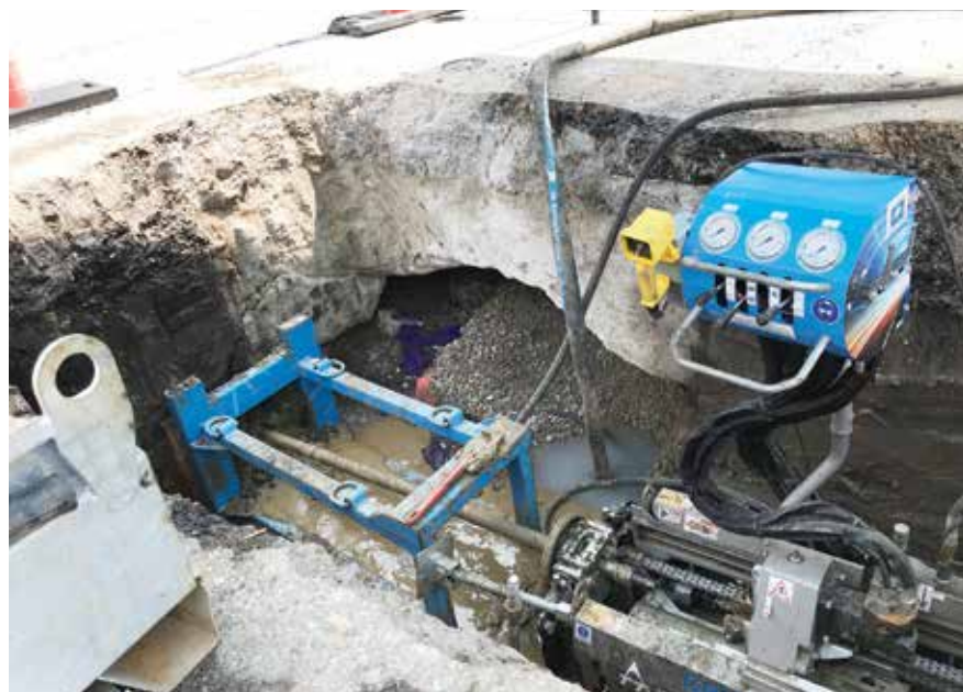
The compact directional drill used by WaterOne measures 54 inches long, 43 inches wide and 57 inches tall; and provides 13,489 lbf of thrust and pulling force
