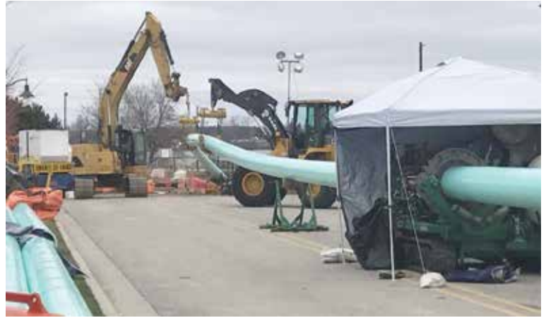
Fusible PVC® pipe entry pit during installation
