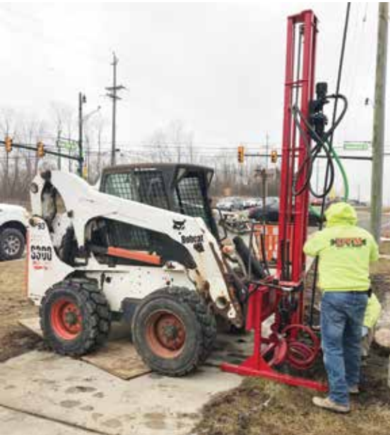
Stand tubes, used to place the stabilizing grout, being inserted
