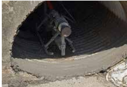
Cement Pipe Rehab
