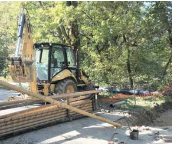
Took patience to work through cobble and hard consolidated clay under the river
