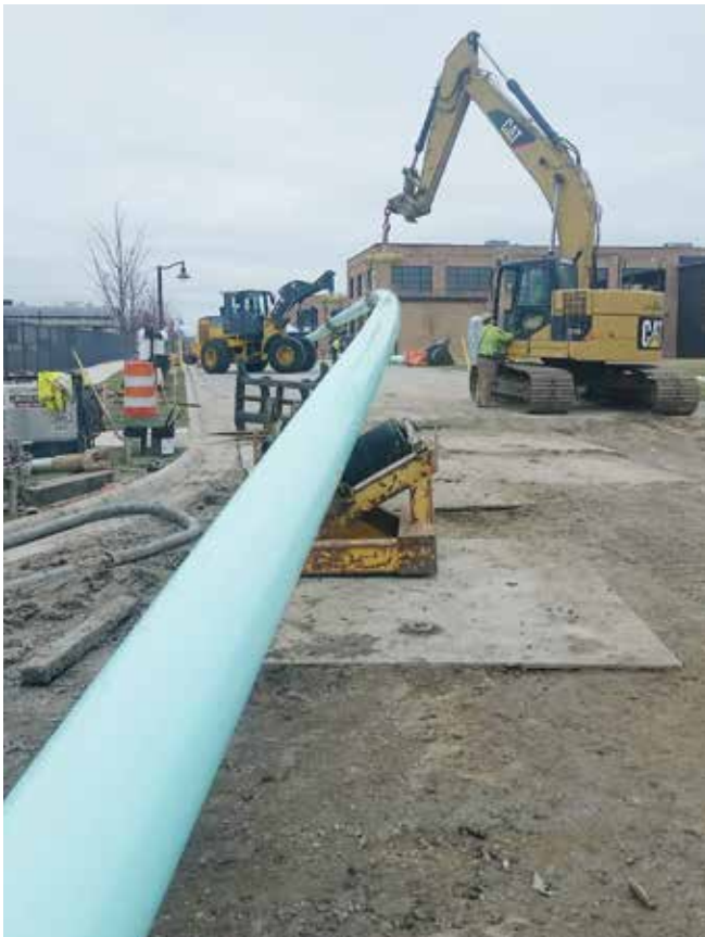
The Fusible PVC® pipe supported on rollers along the alignment
