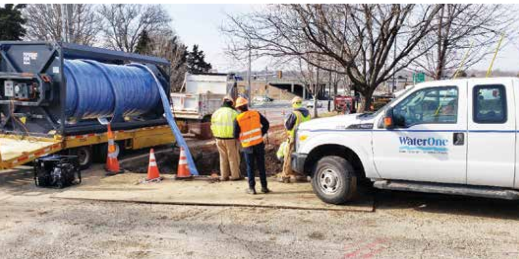
Lining is inserted from a reel, pull-in lasted approx. 3 hours
