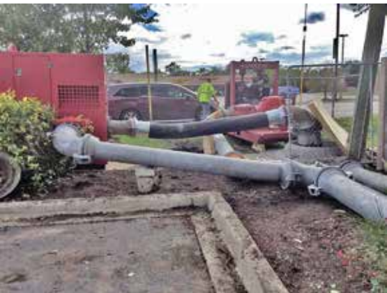
Dual 12-inch pumps were installed to pump all of the upstream flow
