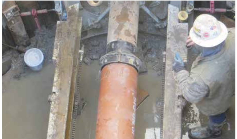
The adapter (expander) fabricated by DVM to manage the jacking forces as the 13 5/16-inch O.D. VCP-J final product pipe was used to push the 11-inch casing out of the bore
