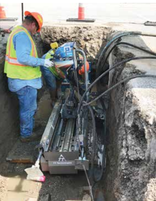
New 12-inch water main needed to be installed under busy street with almost 30,000 cars a day through this intersection. With limited space and other constraints, a compact pit-launched directional drill was chosen for the project
