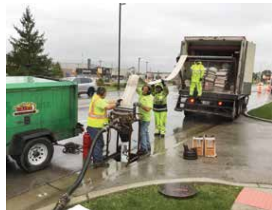
8,200 LF of 8- to 30-inch sanitary sewer was lined over nine days
