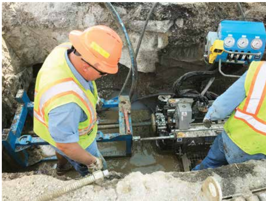
A 1 3/4-inch pilot bore was completed on the first day in approximately 2.5 hours. After reaming, the entire 100-foot, 12-inch PVC line was installed without incident
