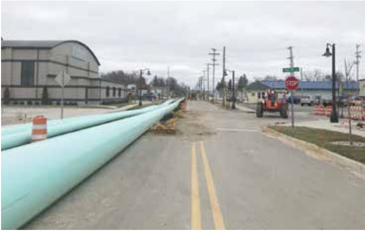
Pipe was staged in 720-foot sections
