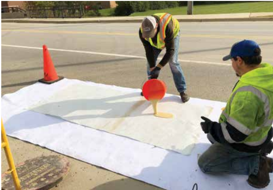
Fiberglass spot liner used to patch hole discovered on final day of lining
