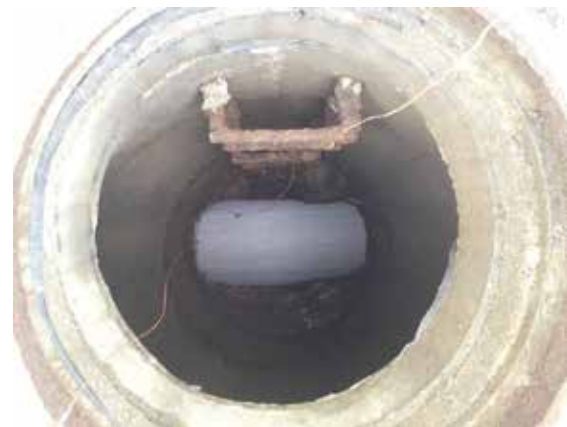
Thirty-one sewer segments were lined in ten "shots" with lining through intermediate manholes
